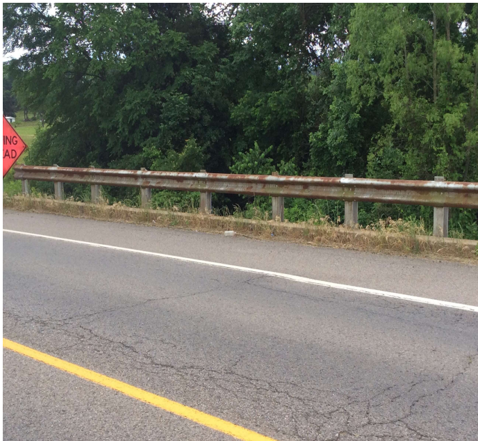
PHOTO 1 Description The paint system is failing with rust showing through the paint.
