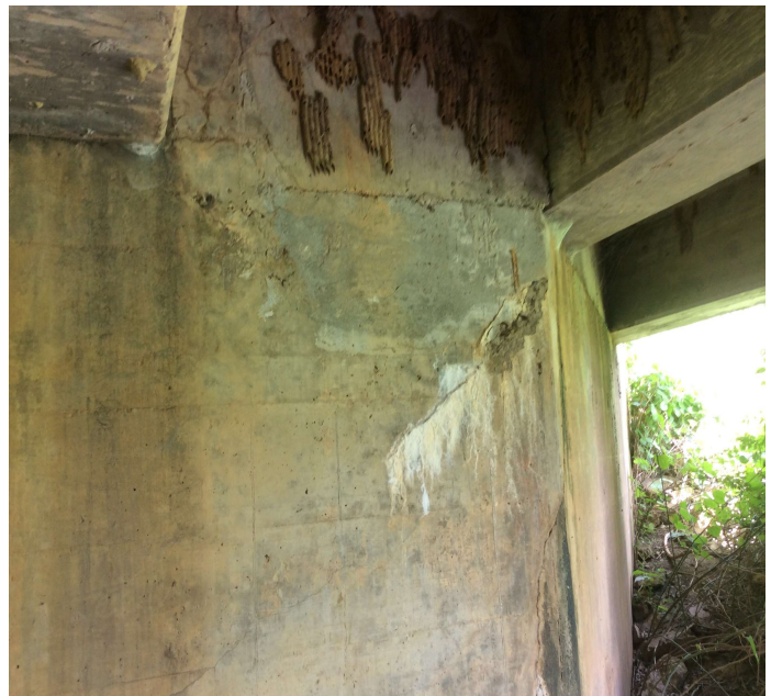
PHOTO 2 Description Bent # 2 RT delaminated area.
