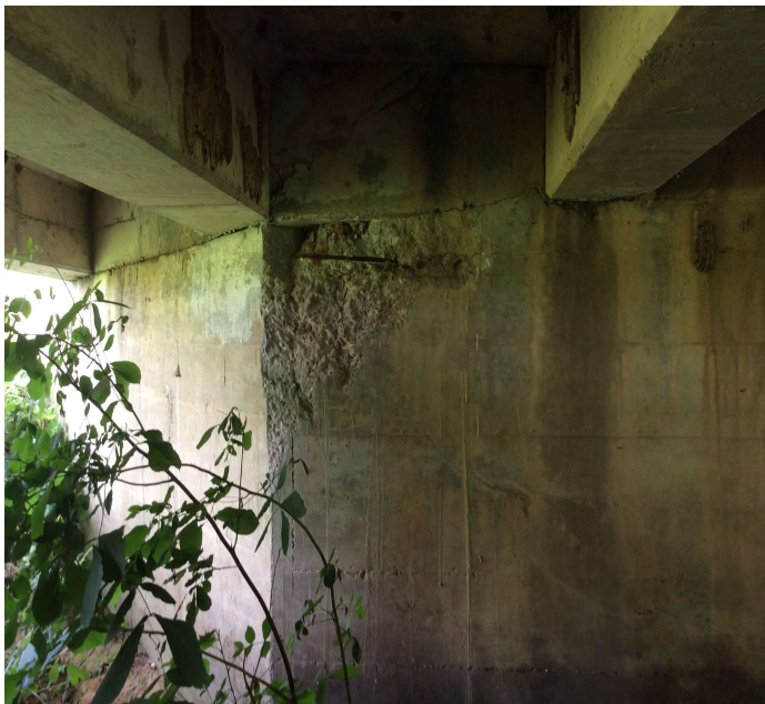
PHOTO 1 Description Bent # 2 Lt spalling with exposed reinforcing steel.
